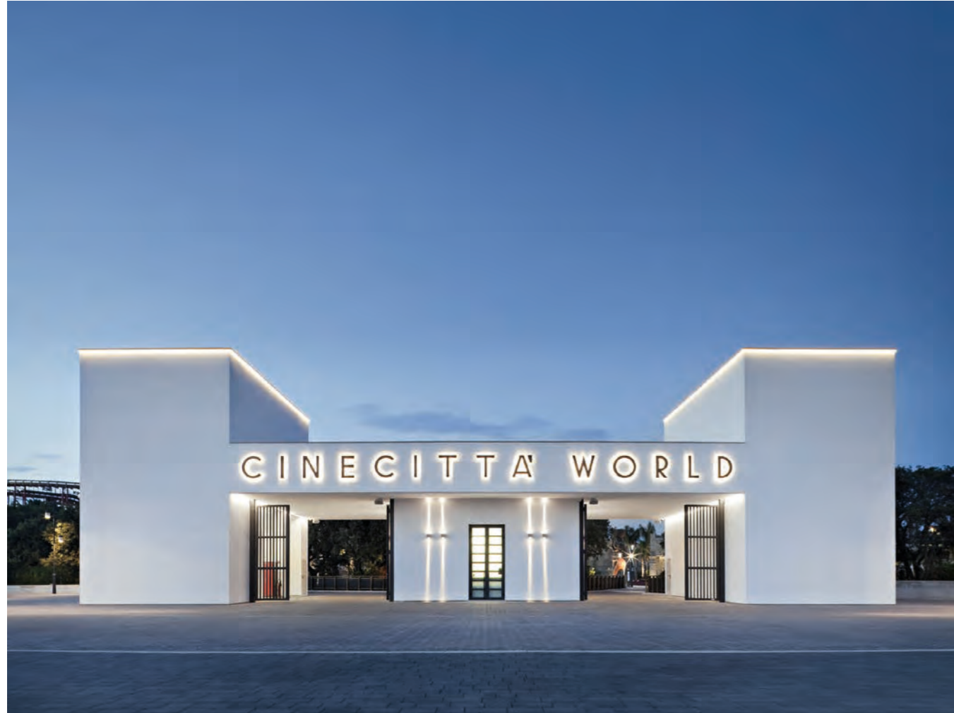
Photographer Germano Borrelli Electrical Engineer Enetec srl
