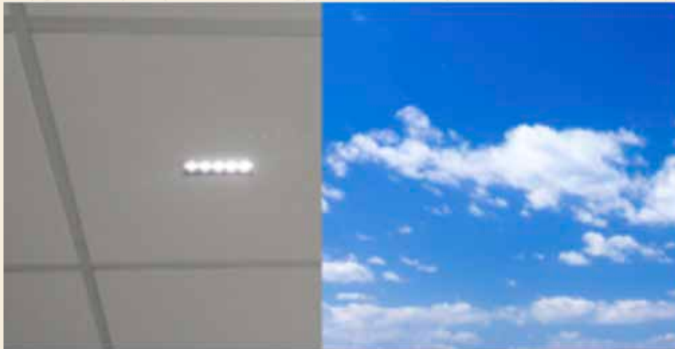
Figure 5. Left: LED ceiling luminaire with high maximum luminance. Right: Northern sky with lower maximum luminance.
